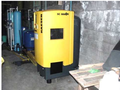
Figura 9: Compresor Airtower 5C
