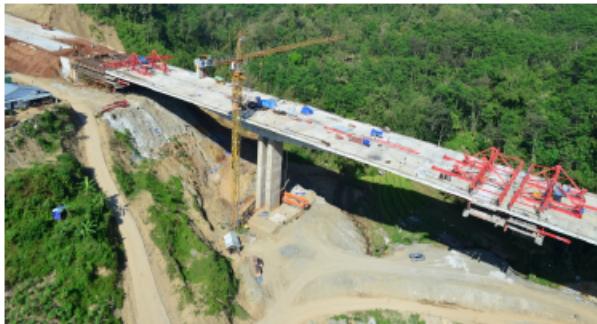
Figura 18: Lemah Ireng II Bridge
