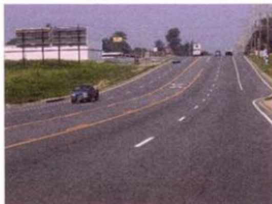
(c) Suburban Multilane Highway Segment with Two-Way Left-Turn Lane
