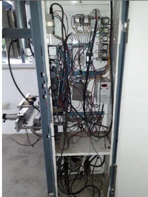
Figura 14: Armario de control
