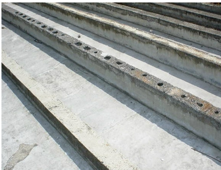
Figura No. 4 Serpentín
