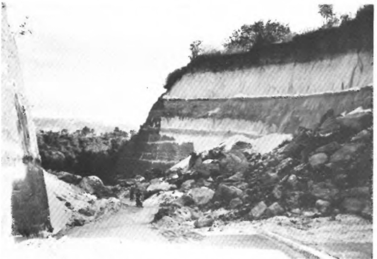
FIGURE 34.—Landslides in steep road cut in stratified pumice and ash deposits at San Cristobal, west of Guatemala City.
