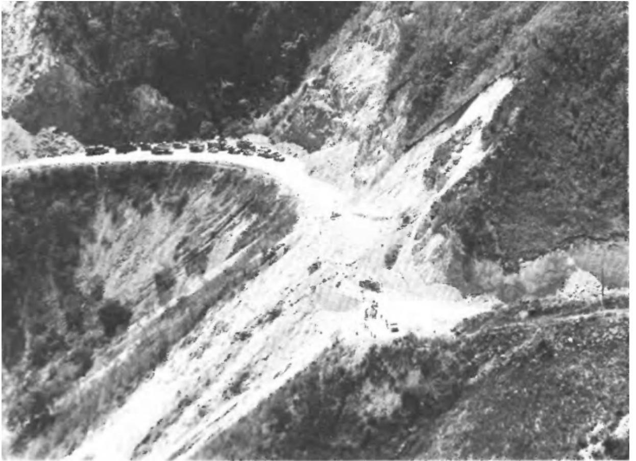
FIGURE 41.—One of the many landslides obstructing the main highway from Guatemala City toward El Progreso.
